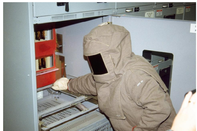
Figure 8 Category 4, 40 cal/cm 2 protection required for this Low-Voltage Circuit Breaker Cubicle work, based on the Flash Hazard Analysis
