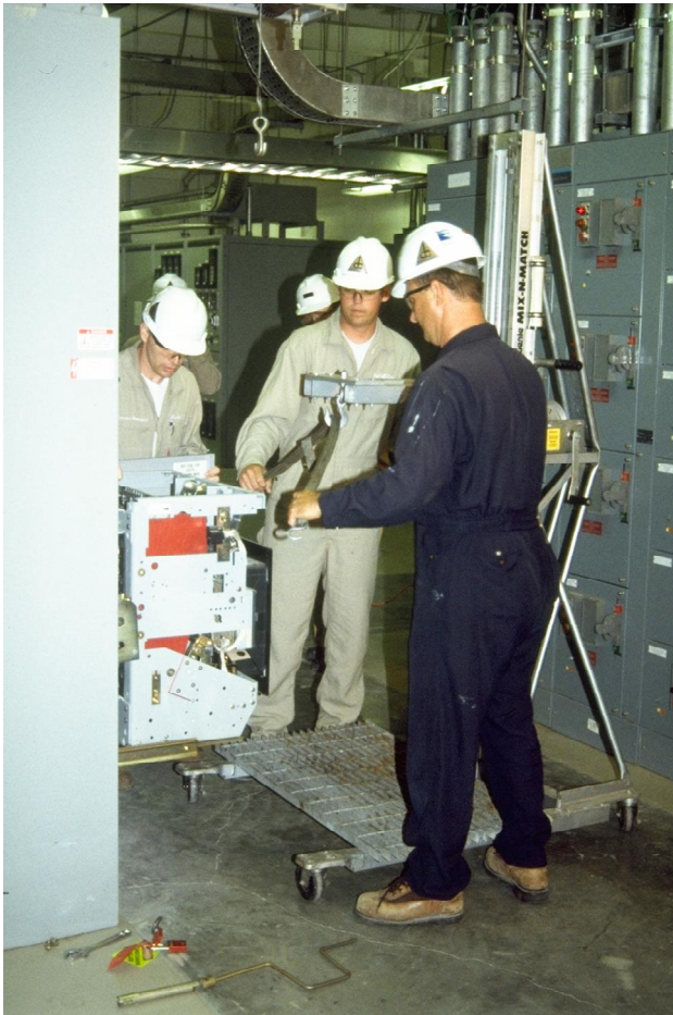
Figure 1 Hands-On Low-Voltage Circuit Breaker Training
